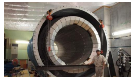
Main Barrel installation (2012 Dec)
